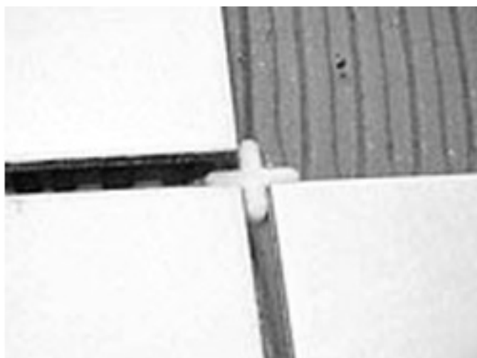
Spacers keep grout width consistent
