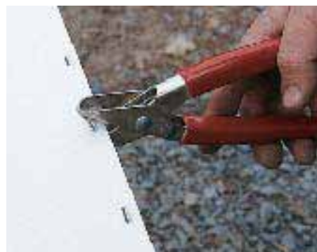
Figure 3. Specialty tools are required for a quality vinyl job. Use a snap-lock punch to make tabs in the top edge of preformed metal fascia (left). These tabs prevent the fascia from pulling out of the utility trim without restricting movement. A slot punch (right) makes the elongated nail holes that allow for movement under a nail head.
