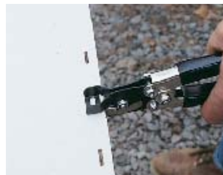
Figure 3. Specialty tools are required for a quality vinyl job. Use a snap-lock punch to make tabs in the top edge of preformed metal fascia (left). These tabs prevent the fascia from pulling out of the utility trim without restricting movement. A slot punch (right) makes the elongated nail holes that allow for movement under a nail head.
