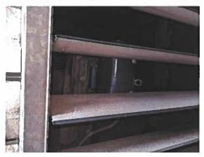
This is the West RTU. The dampers and actuators are in good condition and operational. Edge seals of the dampers are also in very good shape. The return fan visible through the damper appears to be newer within the last 3 years.
