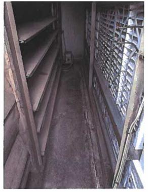
This is the West RTU. The dampers and actuators are in good condition and operational. Edge seals of the dampers are also in very good shape.
