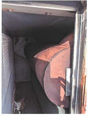
This is the east RTU. The gas burner appears to be in good operating condition.
