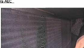
This is the east RTU. This is the other s ide of the cooling coil near the gas burner. It appears to be in very good condition.
