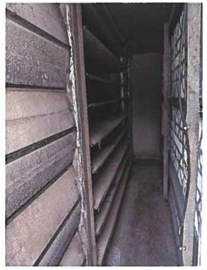
This is the North RTU. The dampers are in good condition. The edge seals on two blades appear to be wearing slightly.
