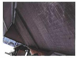
This is the West RTU. The angled condensing coil is in good shape. There are some signs of aggressive pressure washing.
