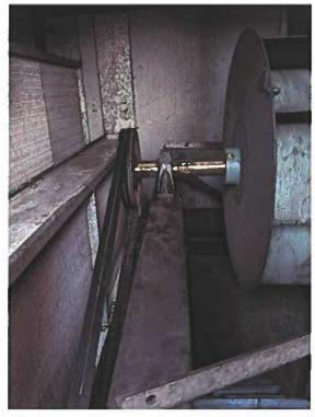
This is the North RTU. The fan bearing was recently greased.
