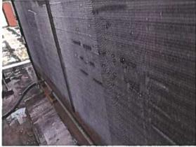
This is the North RTU. The condensing coil appears to be in good shape. There are some signs of writing by a vandal however this should not significantly effect the operation of the coil.
