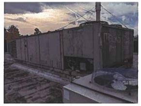
This is the North RTU. The unit has minimal corrosion on the unit housing.
