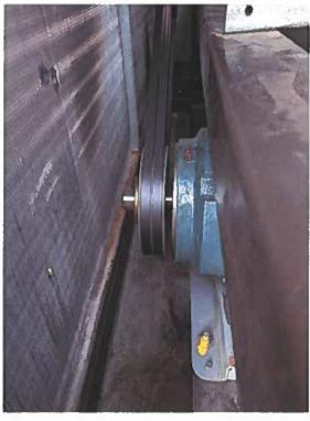
This is the West RTU. The motor bearing appears to have been greased recently.
