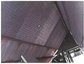
This is the south RTU. The condenser coil appears to be very clean and likely replaced at some point in the life of the unit.
