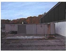
This is the east RTU. The cabinet is in good shape, there is some surface rust near the burner section.
