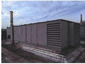
This is the West RTU. There is little corrosion on the body of the unit.
