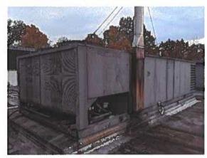
This is the North RTU. The condenser coll is in good condition. The corrosion below the exhaust stack is normal as the flue gases are corrosive and condense on the exhaust stack and are dripping out the bottom of the unit. An acid neutralization kit could be installed and piped to the roof drain to eliminate future corrosion. Also the stainless steel stack should be sealed to the vertical stack riser on the unit.
