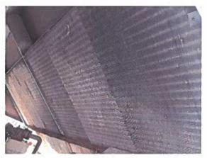
This is the North RTU. The angled condensing coil is in very good shape and appears to be newer.
