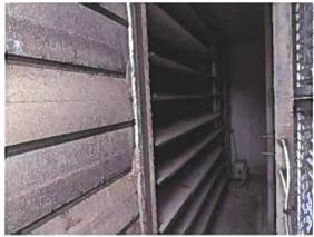
This is the West RTU. The dampers and actuators are in good condition and operational. Edge seals of the dampers are also in very good shape.
