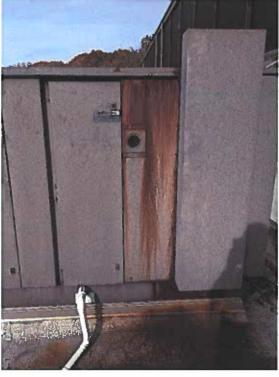
This is the east RTU. The gas burner section has some surface rust.  $\label{eq:continuous} % \begin{subarray}{ll} \end{subarray} % \begin{subarr$
