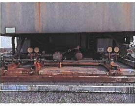
This is the east RTU. This is a view of the compressors. There appear to be no large leaks on this unit.
