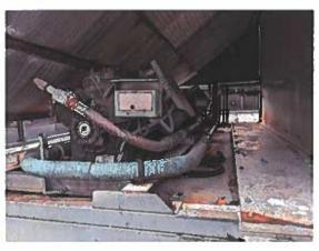
This is the south RTU. The compressor appears to have been replaced at some point. There are no signs of major leaks.
