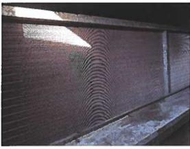
This is the North RTU. The coil inside the unit is very clean, and appears to be newer.
