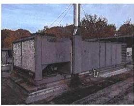
This is the West RTU. There is little corrosion on the body of the unit. The condenser coil is in very good condition. The corrosion below the exhaust stack is normal as the flue gases are corrosive and condense on the exhaust stack and are dripping out the bottom of the unit. A acid neutralization kit could be installed and piped to the roof drain to eliminate future corrosion.
