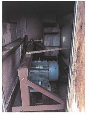
This is the North RTU. The coil, fan and motor are in very good shape. The fan and motor bearings appear to have been greased recently.
