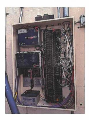
This image shows the main building management control panel for the RTU's. At the time of this photo the controls technician was working on the units.
