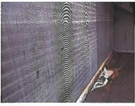
This is the east RTU. This is the other s ide of the cooling coil near the gas burner. It appears to be in very good condition.
