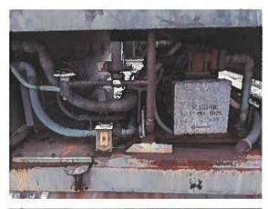
This is the North RTU. The condensers appear to be in operational condition. No major signs of leaks were apparent. A new stainless steel floor plate was installed adjacent to the compressors.
