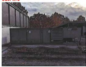
This is the east RTU. The cabinet is in good shape and the unit has a newer louver installed.
