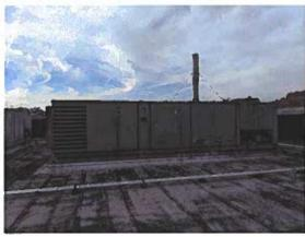
This is the North RTU. The unit has minimal corrosion on the unit housing.
