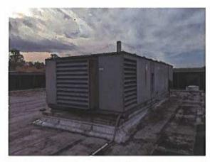
This is the West RTU. There is little corrosion on the body of the unit. A newer louver is visible in this photo.
