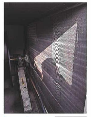
This is the east RTU. The coil appears to be newer and very clean, and possibly replaced within the last 5 or 10 years. The motor and fan bearing were recently lubricated.
