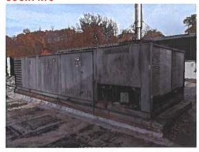
This is the south RTU. There is little corrosion on the body of the unit.
