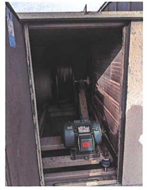
This is the east RTU. The motor appears to be newer and the coil appears very clean, and possibly replaced within the last 5 or 10 years. The motor and fan bearing were recently lubricated.
