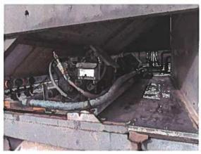
This is the West RTU. The condenser appears to have been replaced within the last 5 years. There are no signs of major leaks. A new stainless steel pan was installed adjacent to the condensers.
