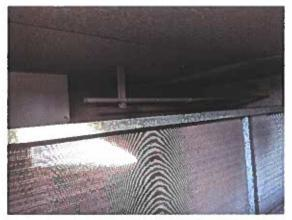
This is the North RTU. The coil inside the unit is very clean, and appears to be newer.
