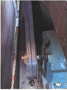
This is the North RTU. The motor bearing was recently greased.
