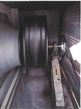
This is the east RTU. The coil appears to be newer and very clean, and possibly replaced within the last 5 or 10 years. The motor and fan bearing were recently lubricated.
