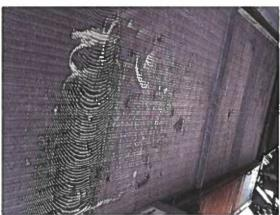
This is the West RTU. The angled condensing coil is in good shape. There are some signs of aggressive pressure washing.
