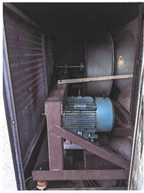
This is the West RTU. The coil, fan and motor are in very good shape. The fan bearing and motor bearings appear to have been greased recently.
