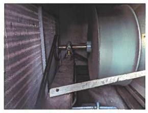
This is the West RTU. The fan bearing appear to have been greased recently.
