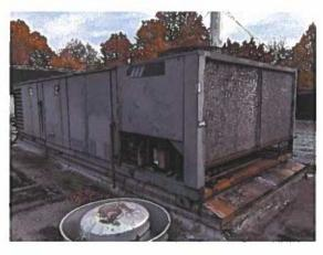
This is the West RTU. There is little corrosion on the body of the unit. The condenser coil has some hall marking but otherwise is in good condition.
